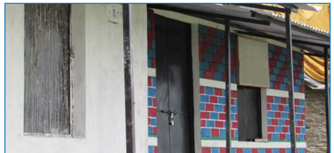
A newly constructed permanent shelter in Yarsha village of Rasuwa district.
