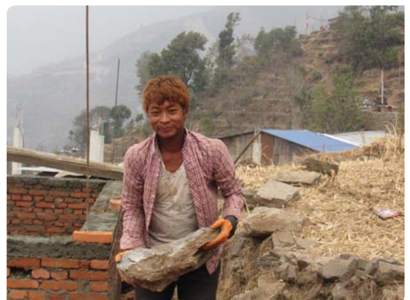
Yudup Thokara works as masons following he was trained on earthquake resistant masonry by LWF and BATAS Foundation.
